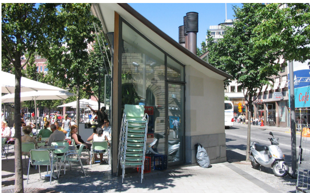
Narrow pavilion units can be developed as a densification typology for places where space is scarce. Stockholm, Sweden
