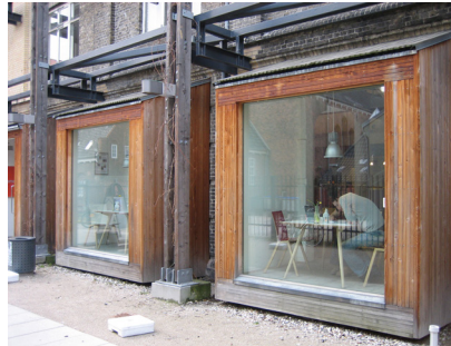
[3] New densification along Rue Erasme with live-work units and active home offices at ground floor, that can be converted to cafés or retail if the retail demand changes.
