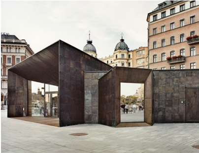
[1] Pavilion programme with visitor information and service as a new face for the Coque towards Avenue J.F. Kennedy
