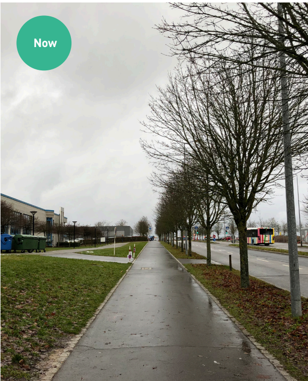
View along Richard Coudenhove-Kalergy to the North and the future Langfuur development. Today a wind-swept and uninteresting walk with no life.
