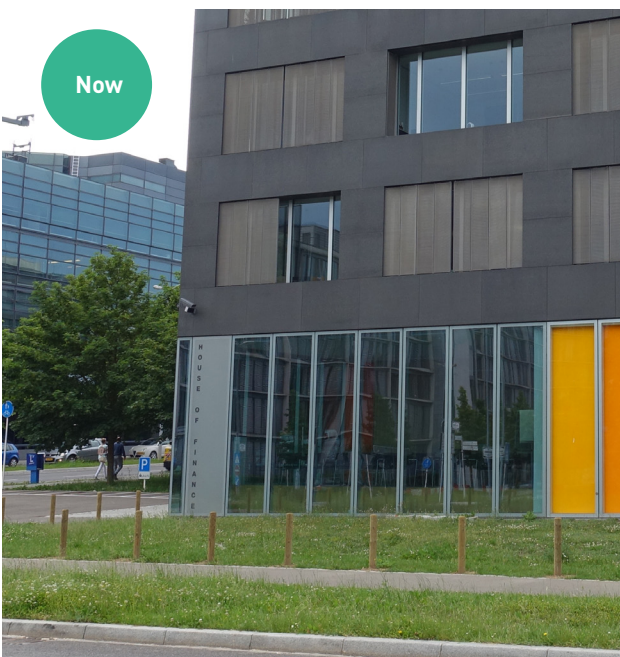
Rue Leon Hengen/Rue Erasme Today an inactive corner in an important, central location that links to the park, d'Coque, and the Roman Way, the central green spine of Kirchberg
